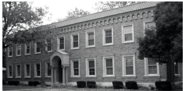
The new Provincial Offices.
